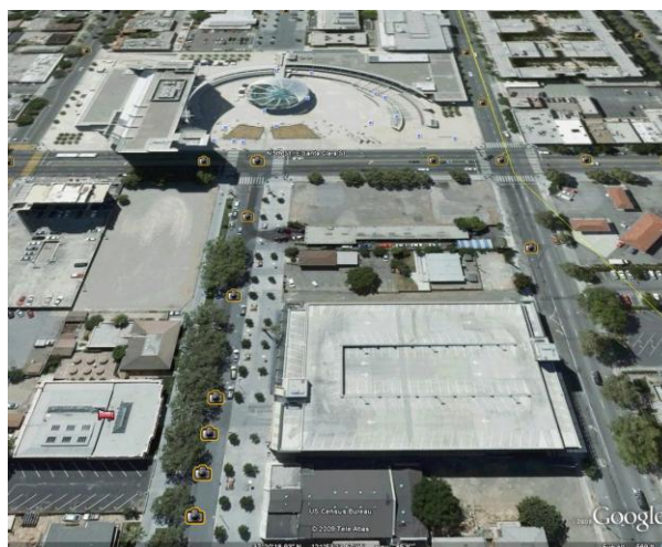
Figure 5-1 7-story parking structure (lower right) serves the 18 story City Hall Tower and complex (upper left)
