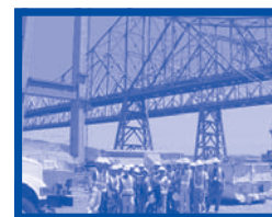
STI students visit the construction site of the new Carquinez Bridge.
