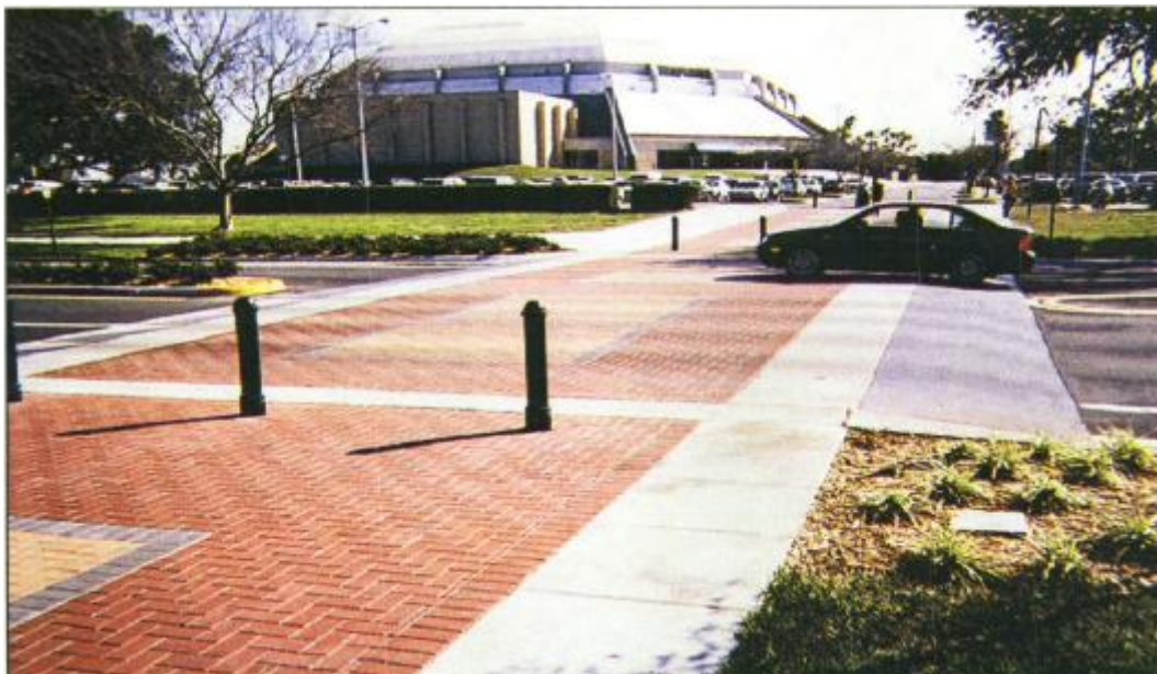
Figure 40. Raised Cross-Walk at Intersection for Pedestrian Safety – Tampa, Florida
