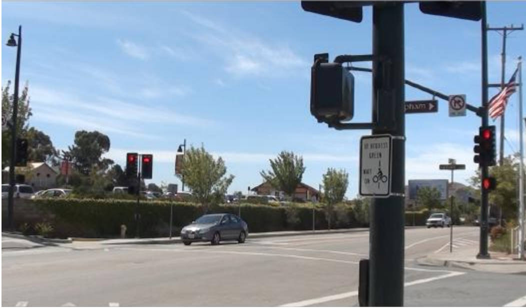
Figure 35. Bicycle Signal Integrated with Auto Traffic Signal– San Luis Obispo, California
