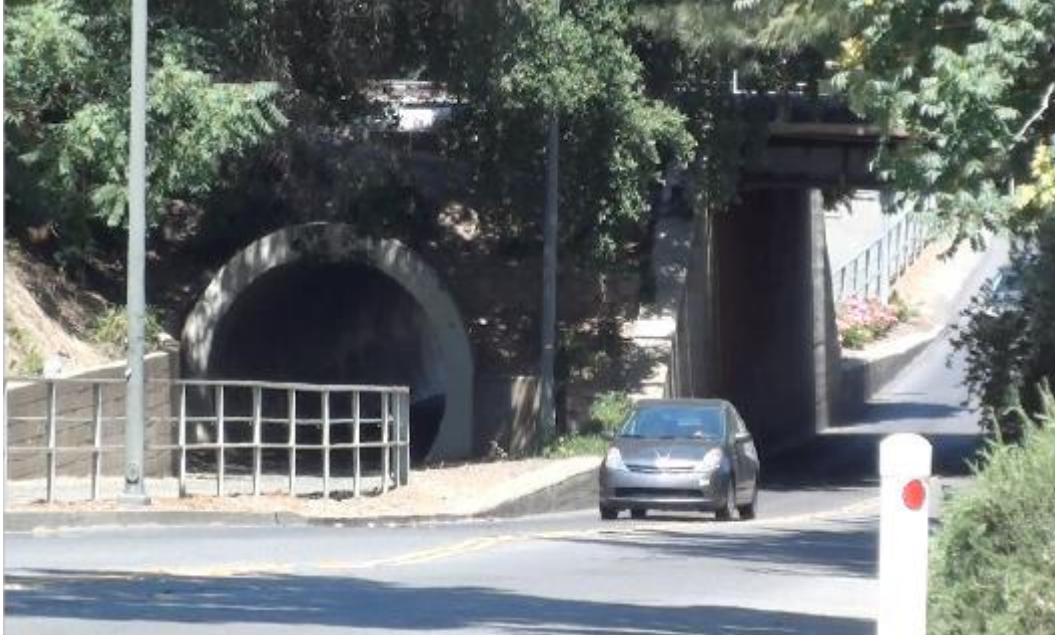
Figure 45. Bicycle Underpass – Davis, California
