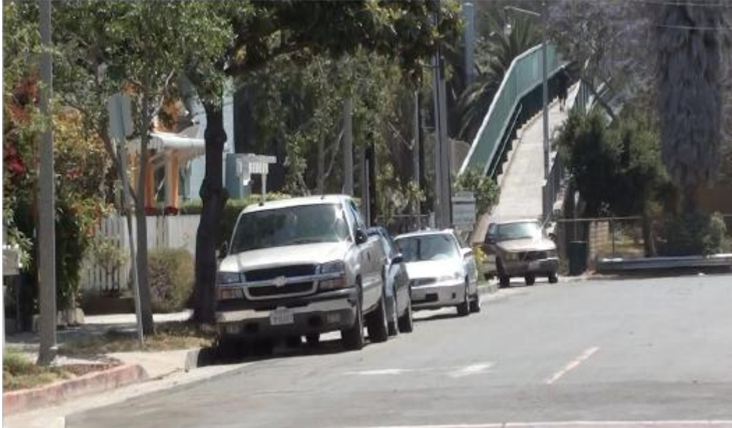
Figure 41. Pedestrian Overpass across US 101 – Santa Barbara, California
