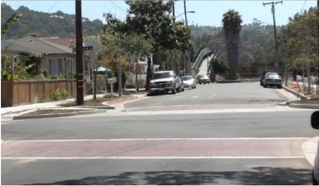
Figure 39. Brick Paving to Demarcate Cross-Walk at Intersection – Santa Barbara, California
