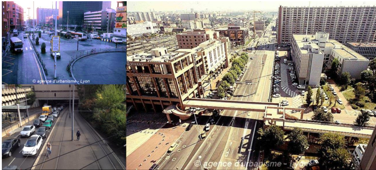
Figure 60. Lyon-Part-Dieu Station 1.0. These views of the Lyon-Part-Dieu station area as originally laid out in the early 1980s show the sol difficile (“pedestrian unfriendly conditions”) surrounding the station. The station area was laid out at the height of the auto-oriented “Les Trente Glorieuses” era, during which the efficiency of automobile circulation was the primary objective of investments in transportation infrastructure. In this initial iteration of the station, pedestrian circulation is one level above the street. As shown in the image lower-left, many pedestrians opt instead to take a more direct and intuitive—albeit dangerous—route along the streetcar tracks, which run parallel to the auto travel lanes. Bicyclists also do this rather than take the more circuitous official bike route around the shopping center. Correcting these poor pedestrian and bicycle connections is one of the key objectives of the current station area redevelopment effort.
