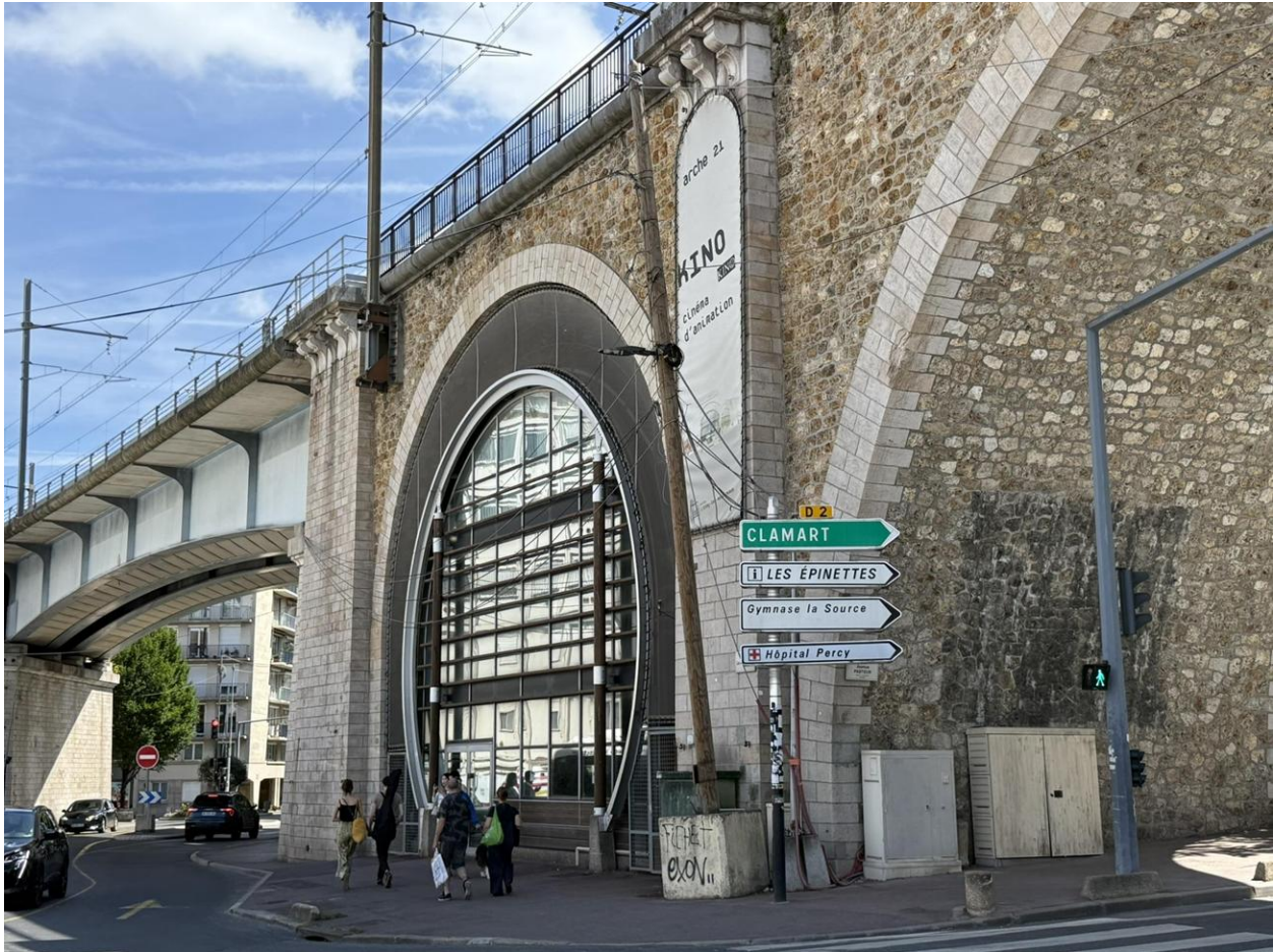
Figure 101. Les Arches at Issy-les-Moulineaux repurposes an old rail viaduct to house artist studios and commercial spaces underneath. The viaduct functions as an active building façade, connecting neighborhoods on both sides while activating previously underutilized urban space.
