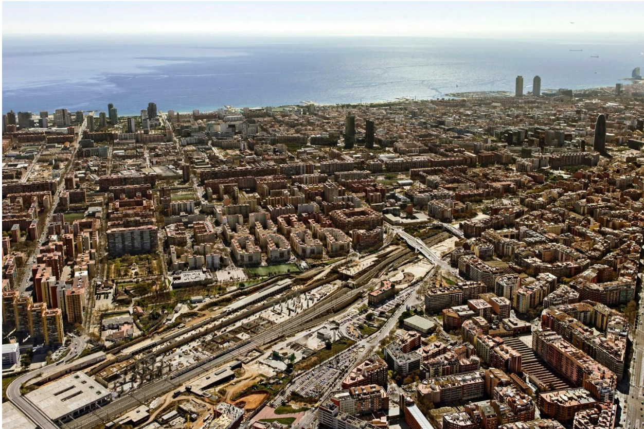
Figure 121. La Sagrera rail yards and construction site.
