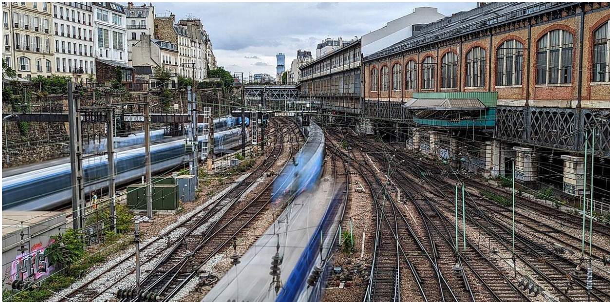
Figure 82. The track approach looking north from St. Lazare. This photo shows how tidily a high-volume and high-capacity rail corridor can fit into a dense urban environment.
