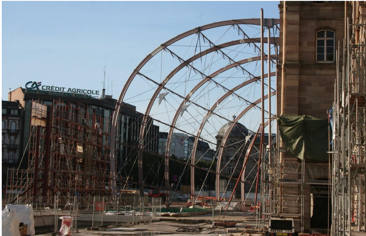
Figure 69. Construction of glass roof.
