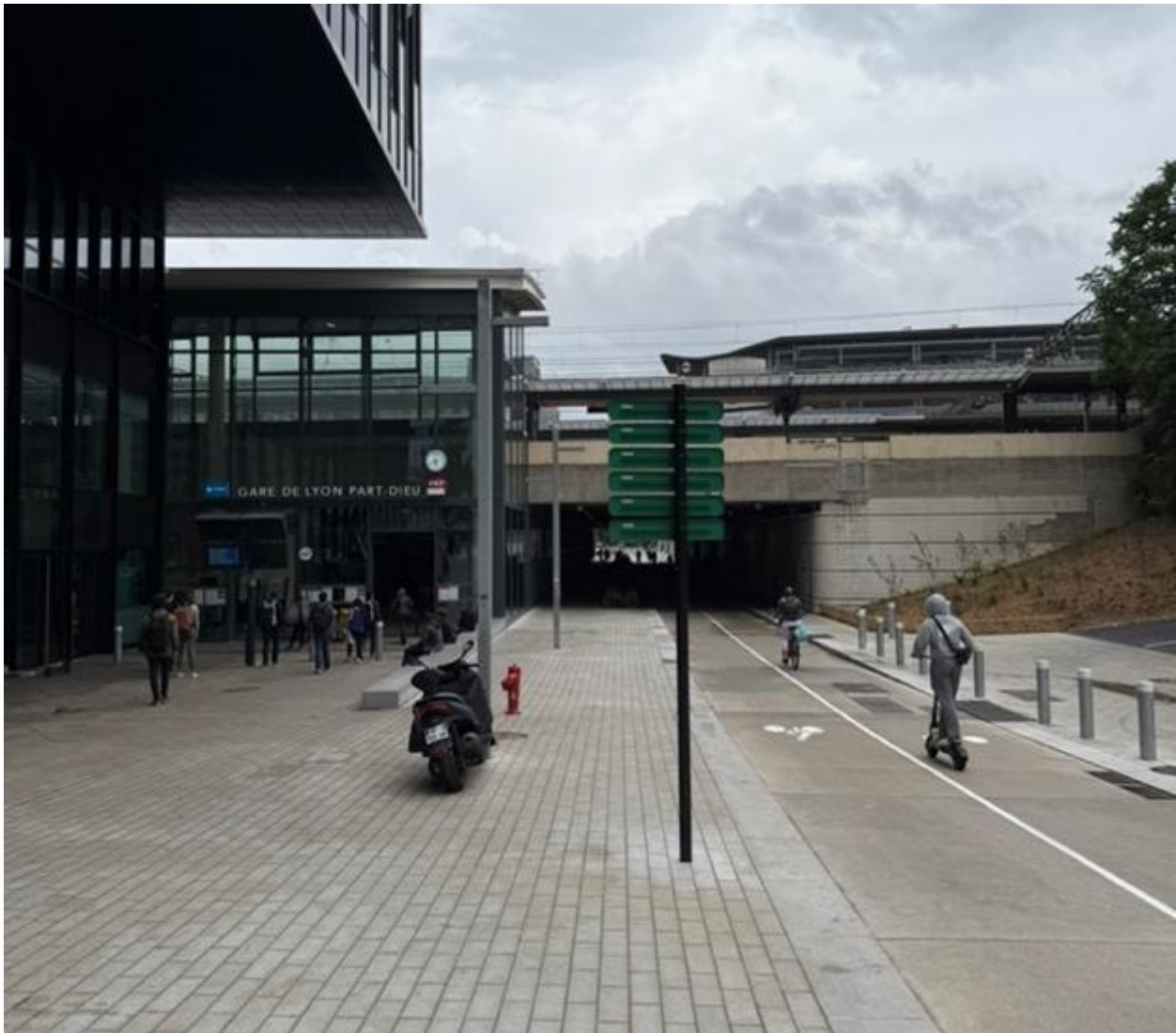
Figure 89. Sidewalk and bikeway leading to the Pompidou Passageway and entrance on the east side of the tracks, facing west. An underpass that used to be for cars, it was slightly reduced in width to make room for the Hall 2 concourse inside the station. Still, even with this resize, there was more than enough room for 13-foot-wide two-way bike lane, and 6.5-foot-wide sidewalks on each side. The station planners turned a thoroughfare for cars into a comfortable crossing for people, taking advantage of a critical access point under the tracks to better connect the two sides.
