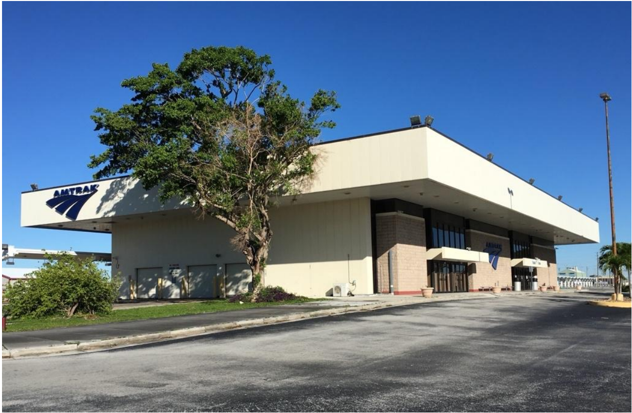
Figure 161. Miami Amtrak Station building. By Phillip Pessar from Miami, USA - Amtrak Station Hialeah, CC BY 2.0, https://commons.wikimedia.org/w/index.php?curid=64176007
