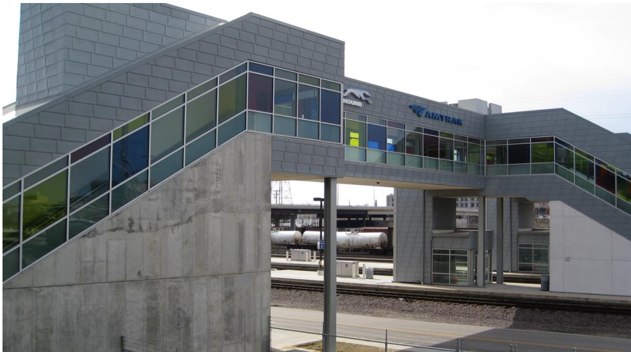
Figure 154. Track access at St. Louis Gateway Station. The utilitarian design necessitates a significant vertical transition for passengers, requiring them to ascend and descend to cross the tracks. Unlike many European models studied, the station acts as a physical barrier rather than a multi-modal connector for the surrounding neighborhood.
