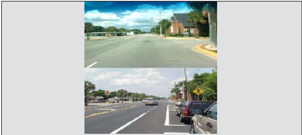
Figure 2. Edgewater Drive, Before and After Restriping.
