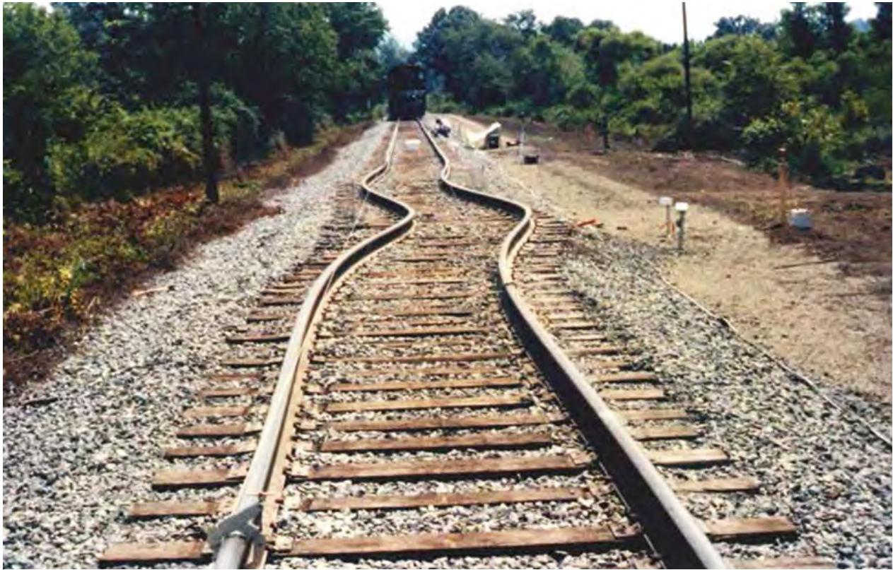
Figure 10. Buckled rail (sun kink) from extreme heat. Source: NOAA, 2017.
