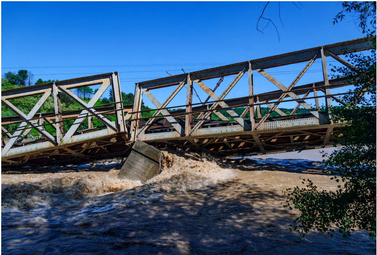
Figure 5. Railroad bridge with flood damage. Source: Adobe Stock
