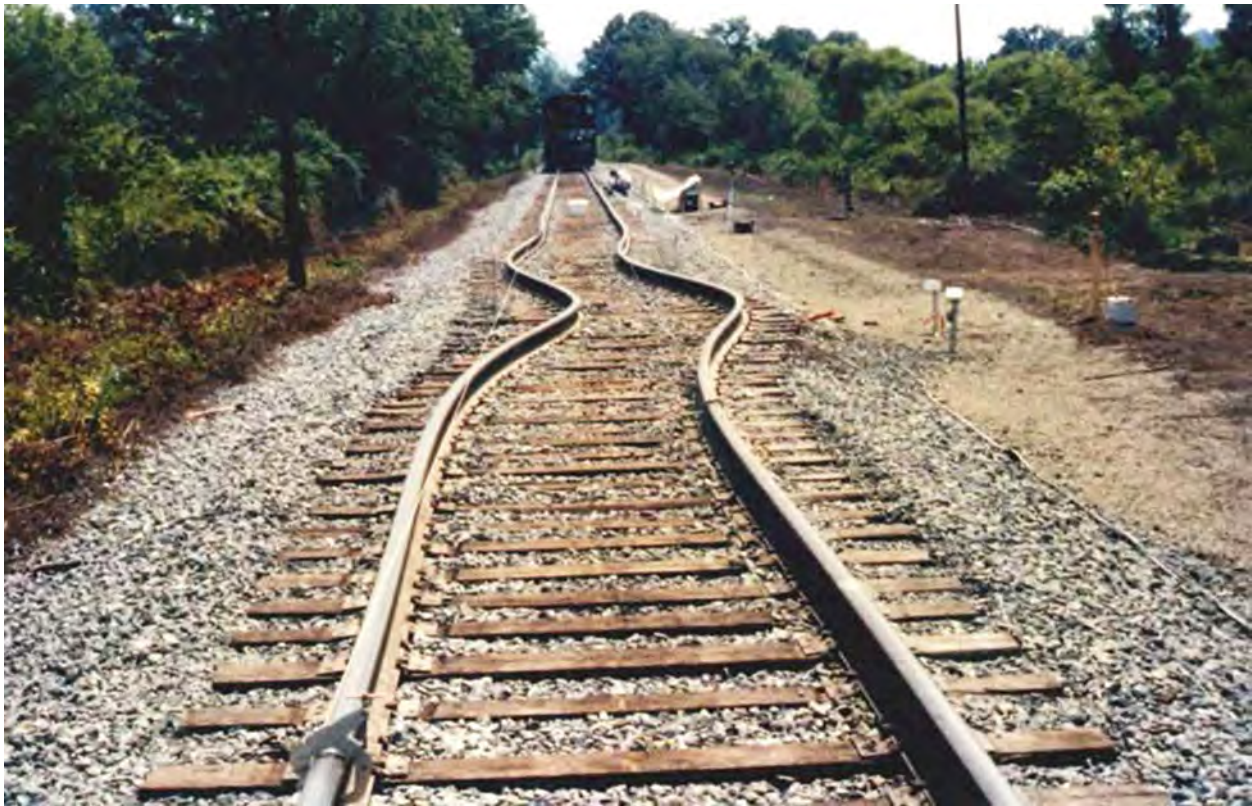
Figure 2. Buckled rail (sun kink) from extreme heat
