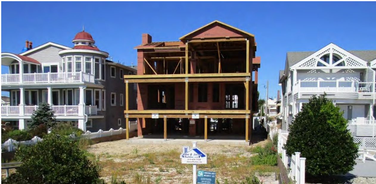
Figure 13. New construction to post-Sandy building code in Ocean City, New Jersey
