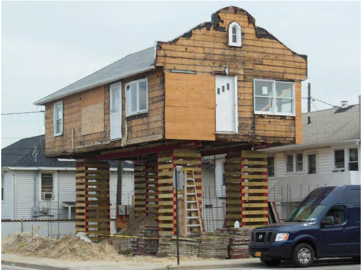
Figure 12. House being raised in Long Island, New York
