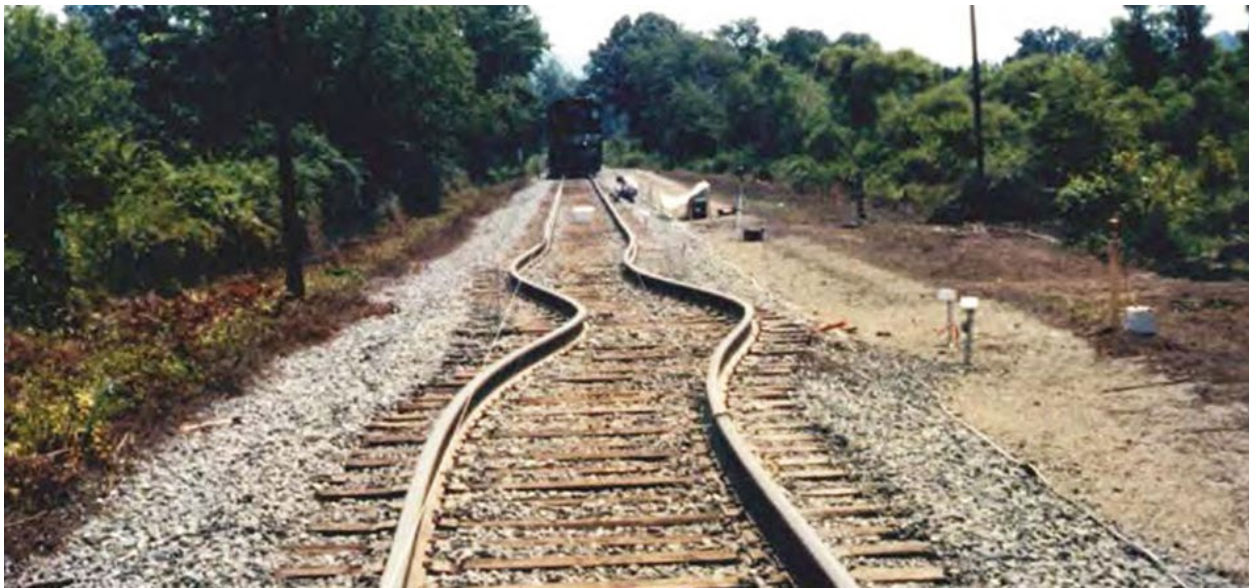
Figure 3. Buckled Rail (Sun Kink) from Extreme Heat
