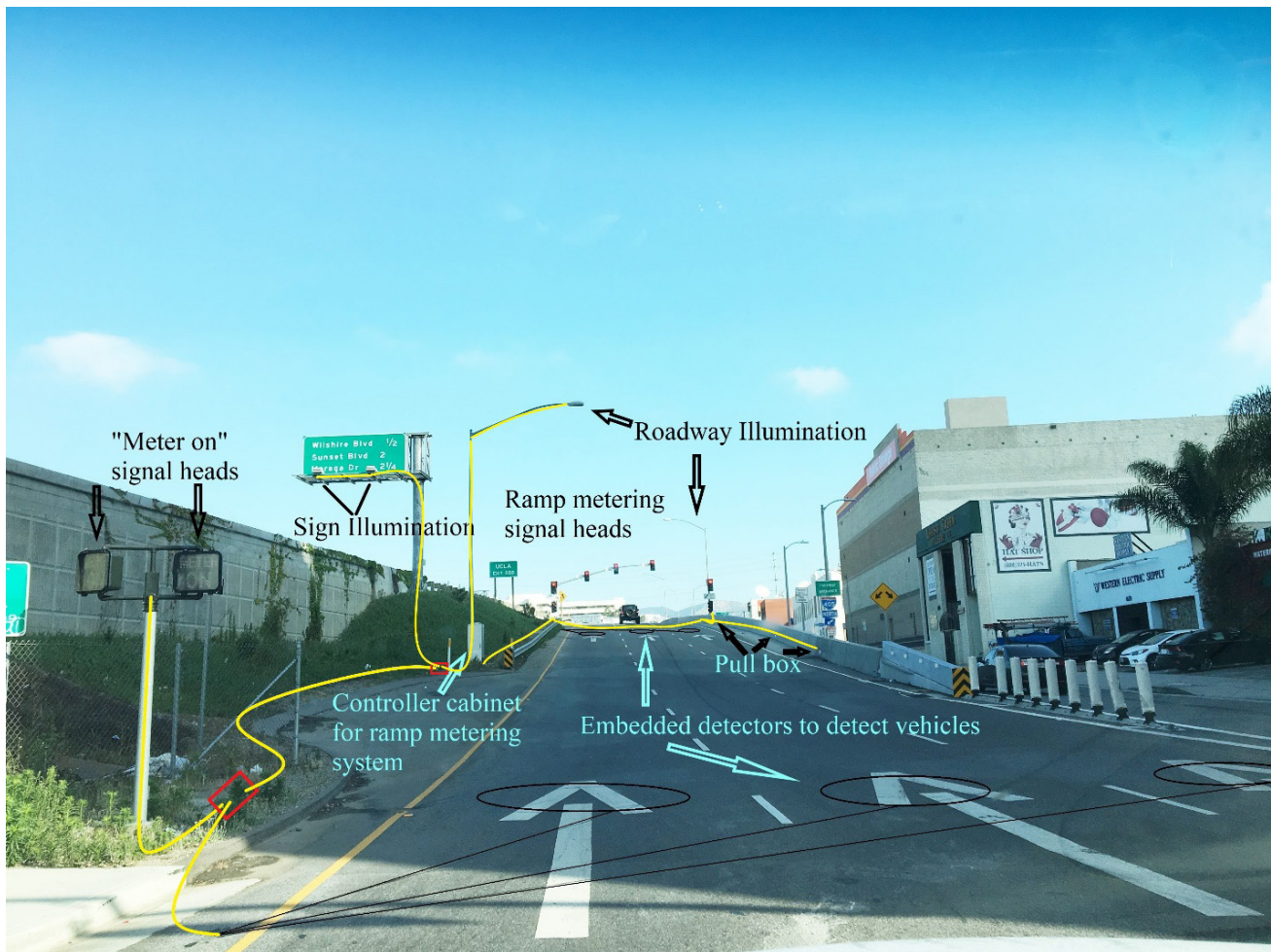
Figure 2. Illustration of Copper Wire Use in Roadways -- Santa Monica Blvd on-ramp to Route 405 northbound. Yellow lines represent copper wire in the infrastructure.
