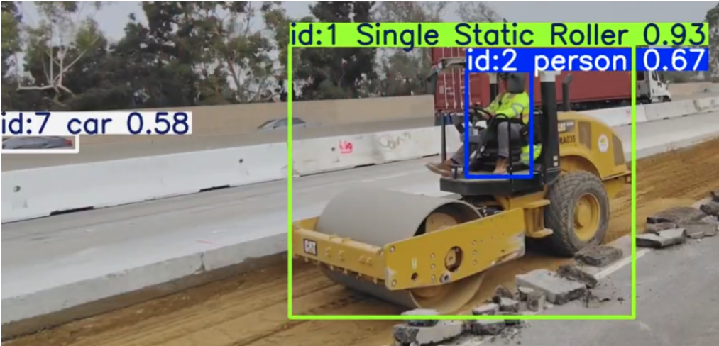
Figure 5.3. Sample Output for a Highway Construction Site
