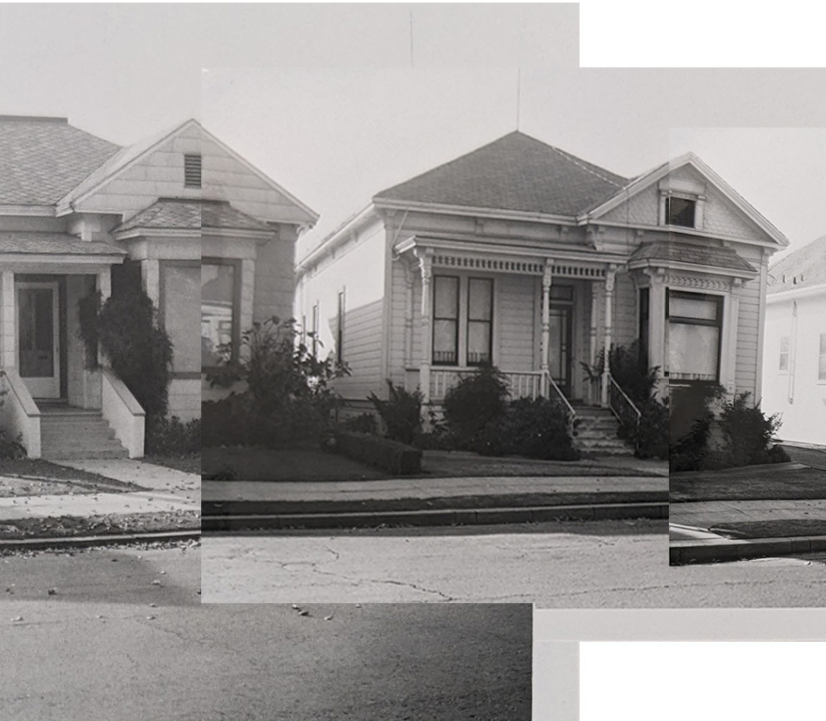
A composite photo created to show a street-level, mid-block perspective of homes that were demolished. L to R: 451, 449, and 441 Delmas Ave. Original photos from Caltrans Right of Way Assessments 1960 - 1970 archival collection, San José Public Library.
