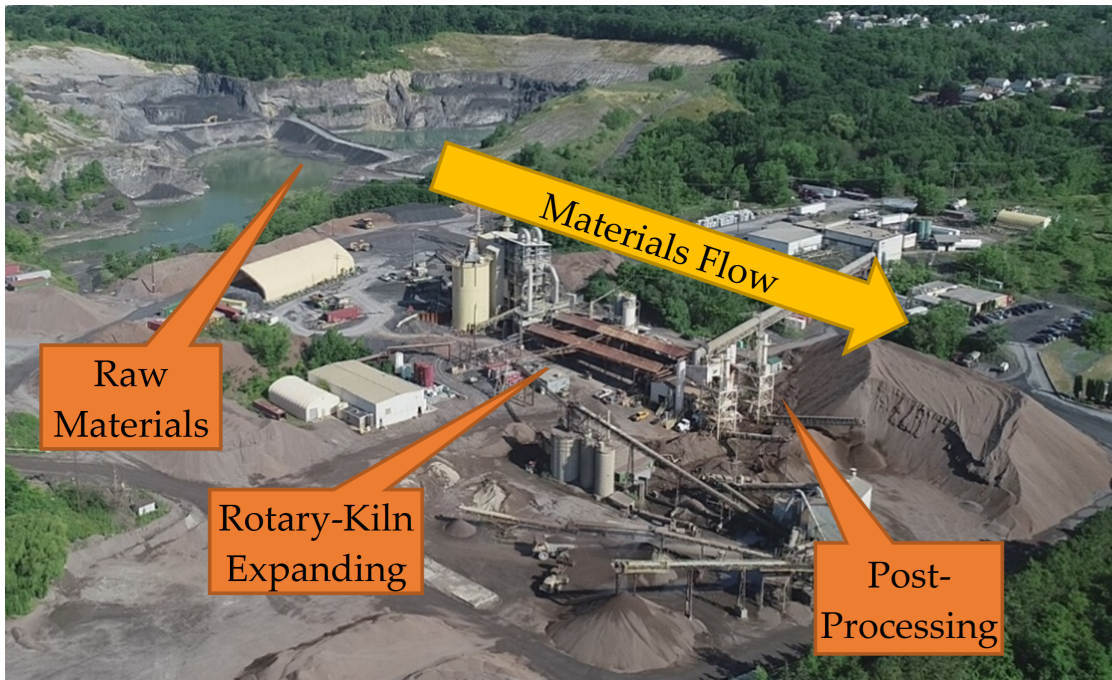
Figure 4. A Rotary-kiln Manufacturing Plant of Expanded Aggregates (Courtesy of Norlite)
