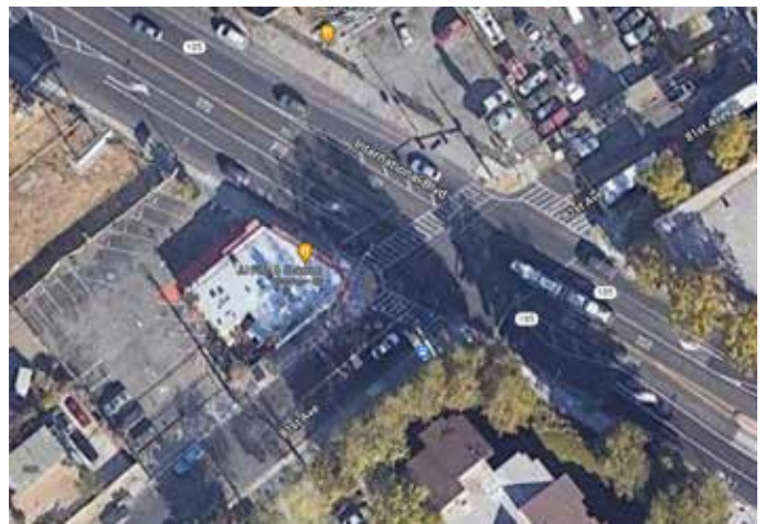
Missing crosswalk on south leg of intersection with 81st Avenue, on the Allen Temple Arms side of the block.
