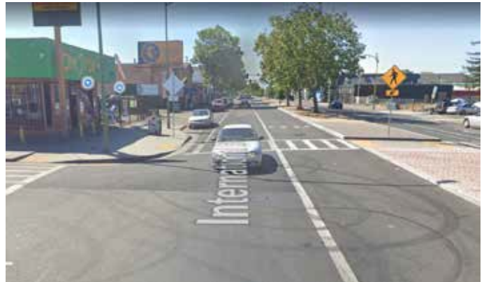
Crossing at One Stop Market is well marked, but only has signage alerting motorists of pedestrians instead of something more visible such as a flashing beacon.
