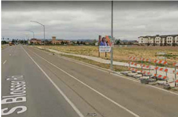
Blosser Road's wide ROW includes a center median and sidewalks, bike lanes on each side.
