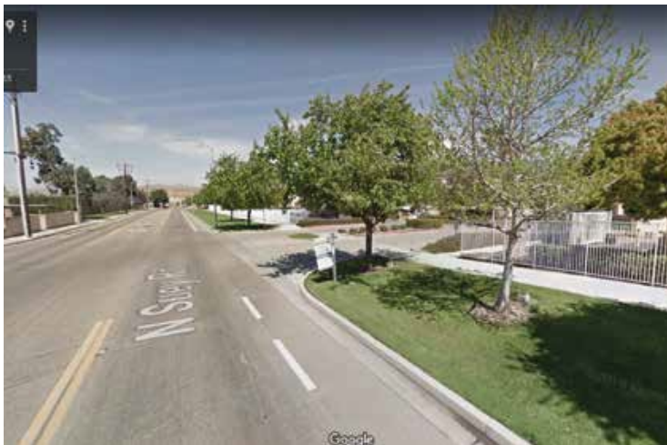
Entrance seen via Google Street View
