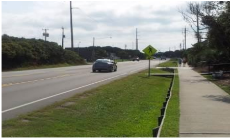
Sidepath next to 2 motor vehicle lanes, CLTL
