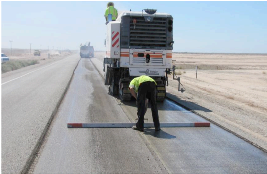
Figure 61. Micro-milling Operation (Courtesy P.R. Systems, Inc.)
