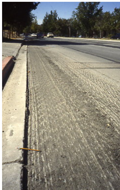
Figure 57. Edge Milling/Key Cutting
