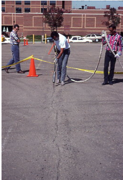
Figure 8. Air Blasting of Routed Crack (Courtesy of CrafcO)
