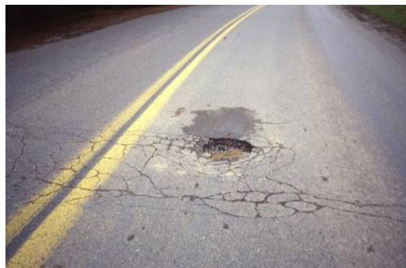
Figure 30. Typical Pothole
