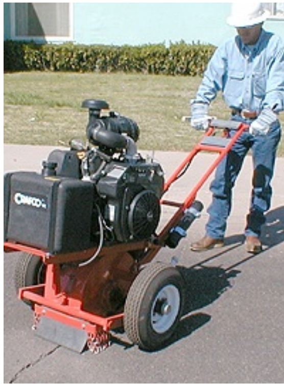
Figure 18. Routing to Create Crack Reservoir
