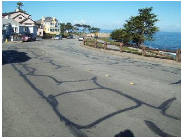
Figure 2. Ugly Crack Sealing on a Scenic Street
