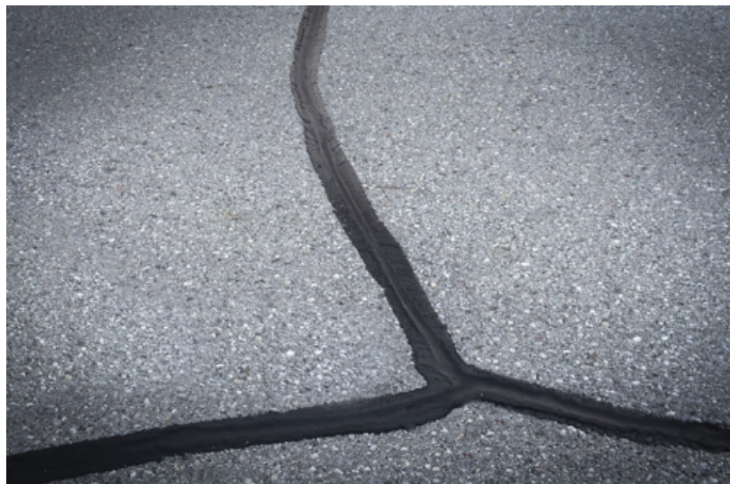
Figure 15. Good Overband Method (Courtesy of Roger Smith, 2021)
