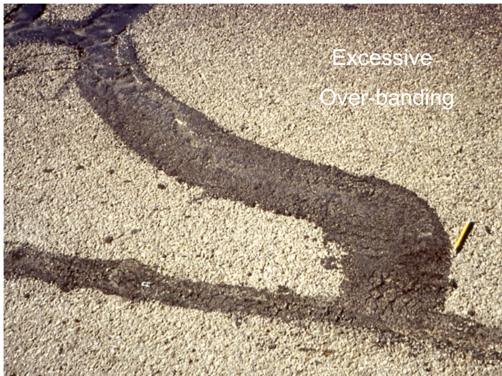
Figure 16. Excessive Overband
