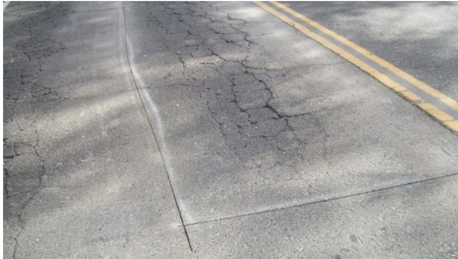
Figure 35. Marked Cut Lines for Small Digout
