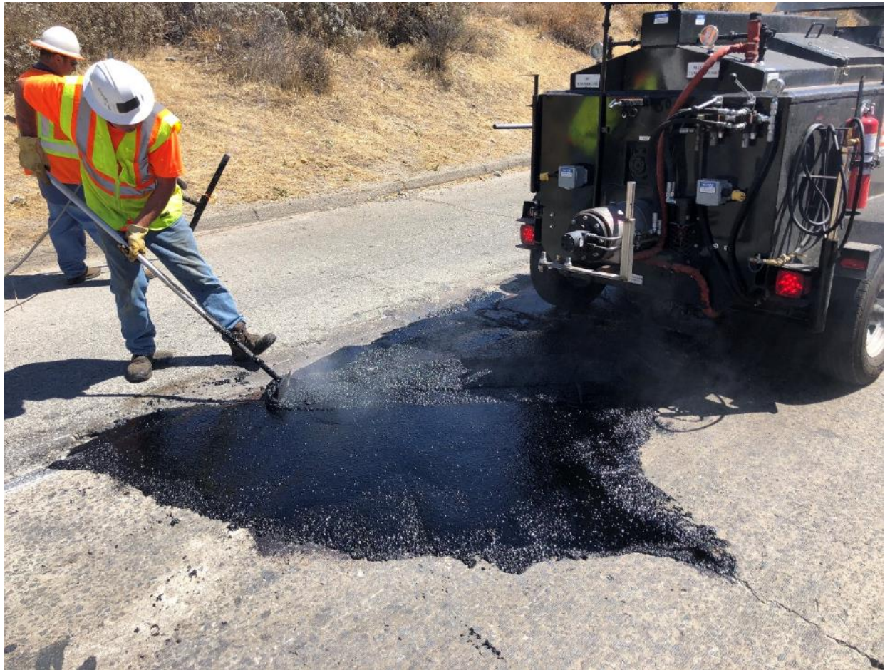
Figure 43. Hot Mastic Patching (Courtesy of Maxwell)
