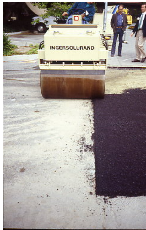
Figure 38. No Vibratory Rolling on Surrounding Good Pavement
