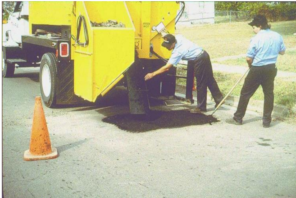
b. Unload Patching Material from Patching Truck
