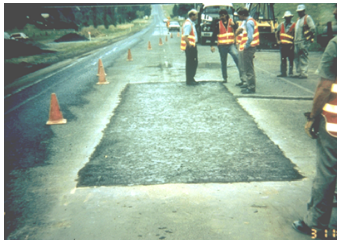
Figure 39. Completed Digout Patch using HMA (Caltrans MTAG, 2009)
