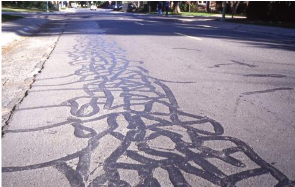
Figure 3. Attempt at Sealing Alligator Cracking
