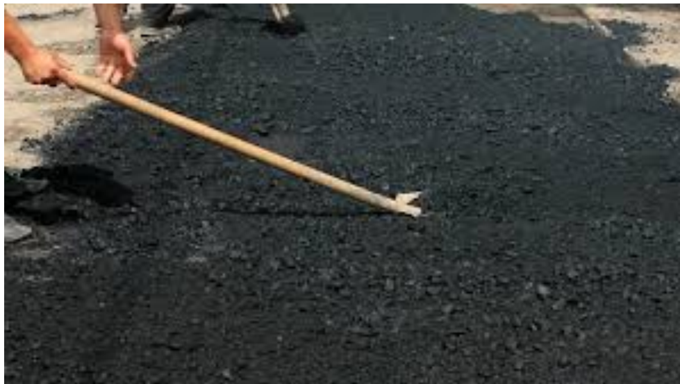
Figure 49. Hand Leveling of a Skin Patched Area
