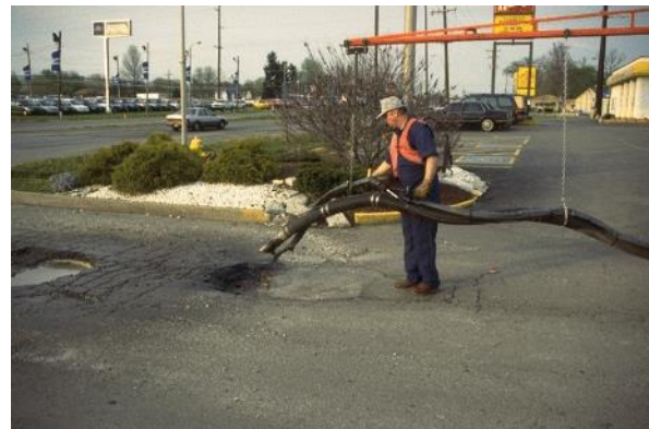
b) Application of Tack Coat
