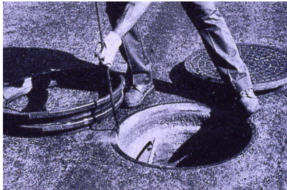
a. Clean Up Existing Manhole Ring & Cover
