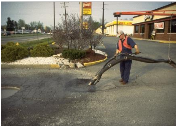
c) Filling the Prepared Hole with a Mixture
