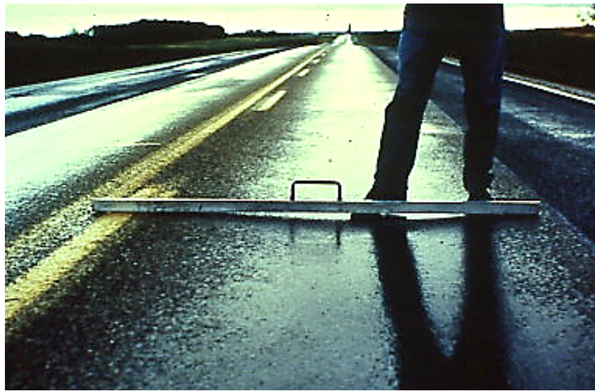
Figure 62. Rutting Requiring a Leveling Course Prior to Overlaying
