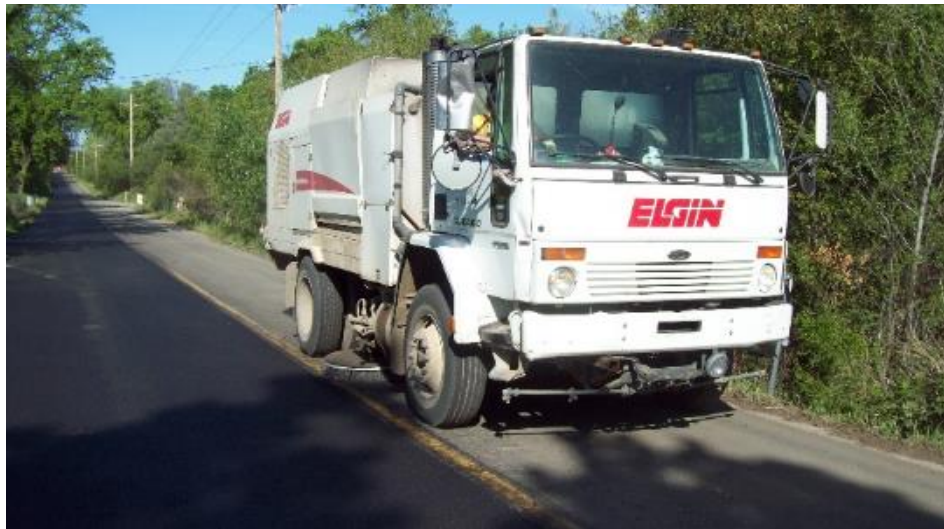
Figure 52. Sweeping Prior to Resurfacing
