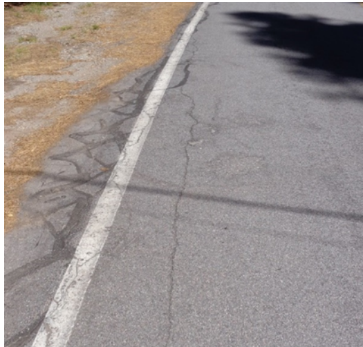
Figure 51. Example of Edge Cracking of a Pavement
