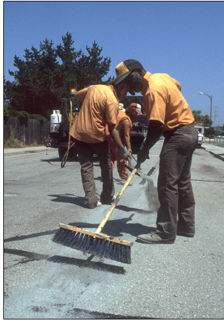
Figure 22. Brooming Blotter Coat over a Treated Crack
