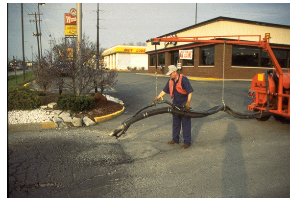
d) Application of Finish Coat of Aggregate
