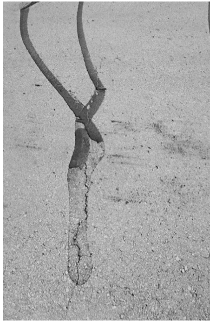
Figure 12. Sealant Peeling as Result of Improper Cleaning (Courtesy of CrafcO)
