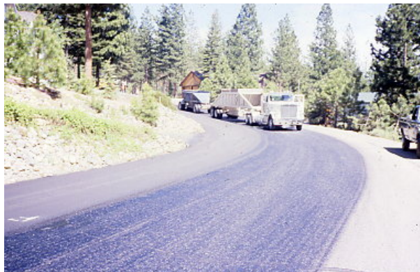
Figure 55. Sparse Tack Coat after Break
