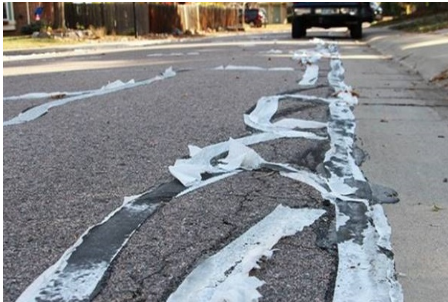
Figure 23. Improper Blotting Techniques Using Paper
