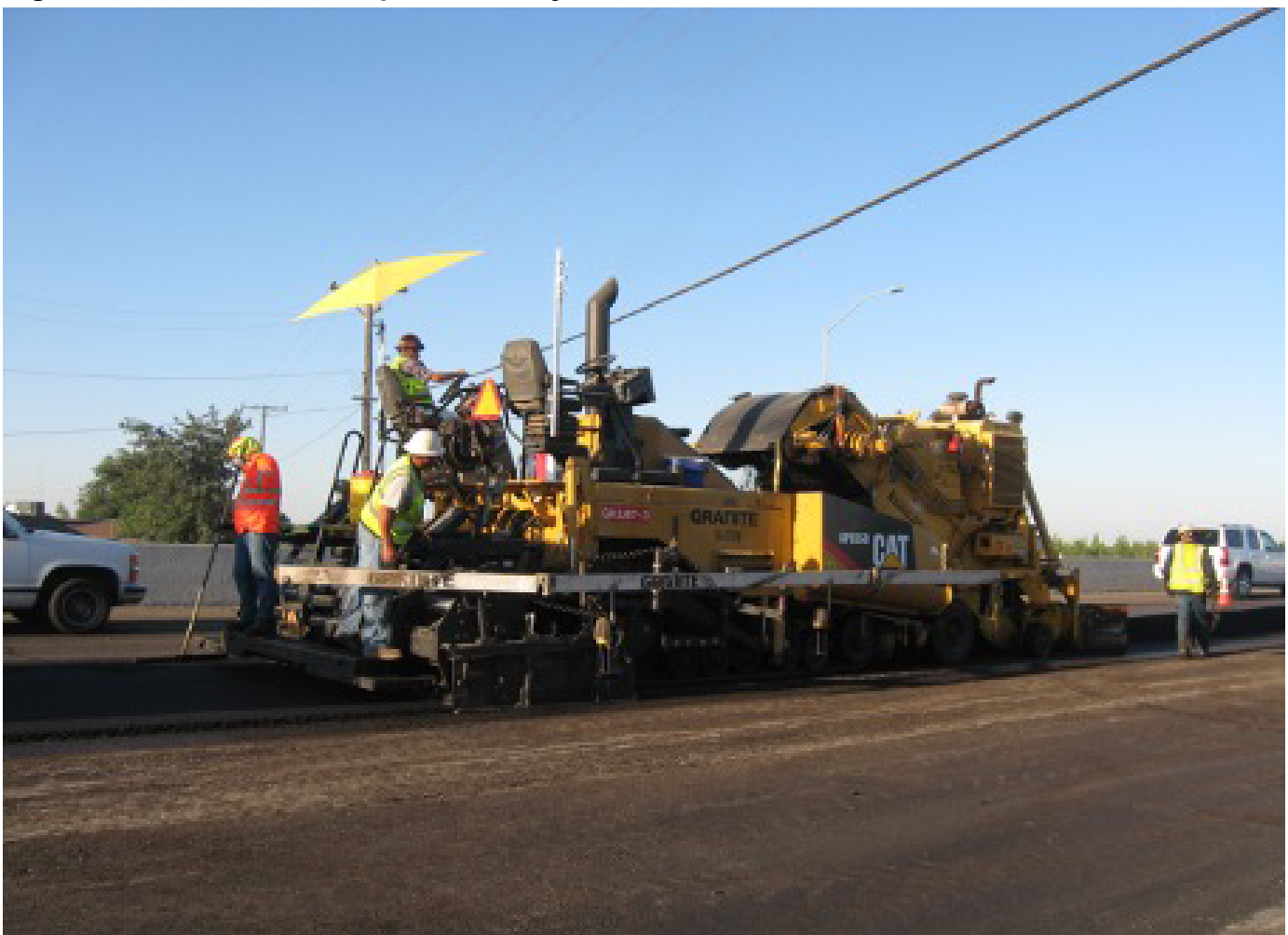
Figure 4. Thin Hot Mix Asphalt Overlay Construction
