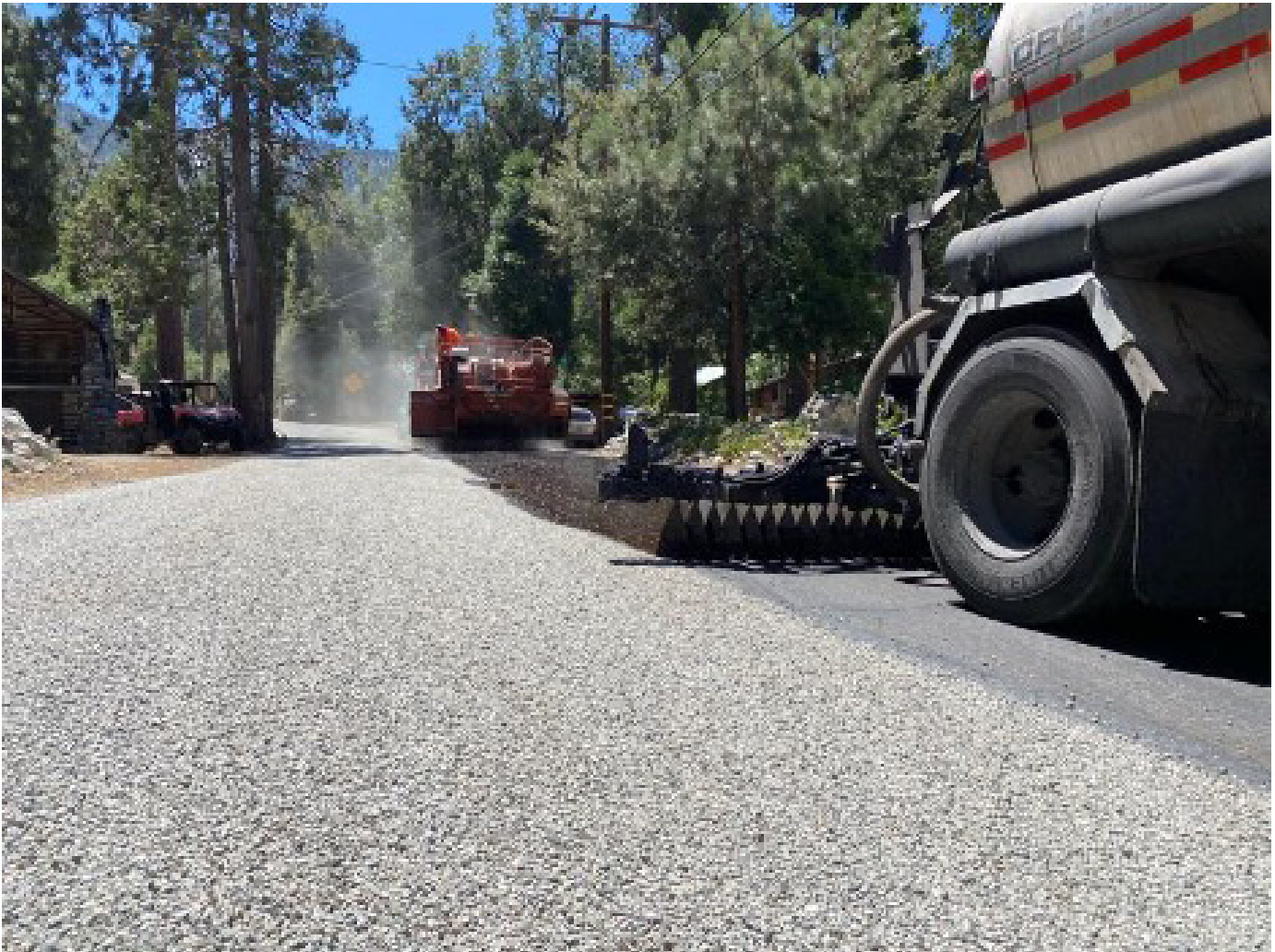
Figure 1. Typical Chip Seal Operation
