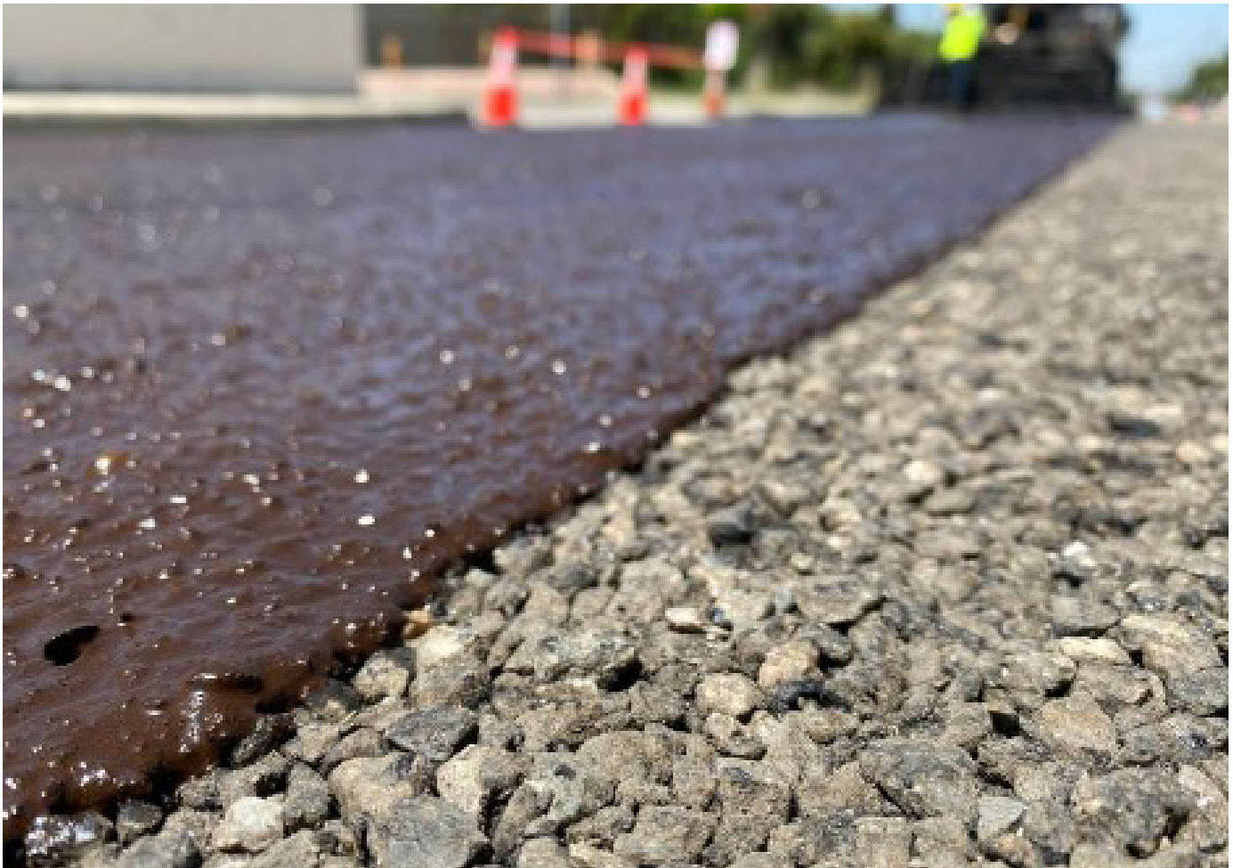
Figure 3. Completed Cape Seal—Slurry Seal over Chip Seal
