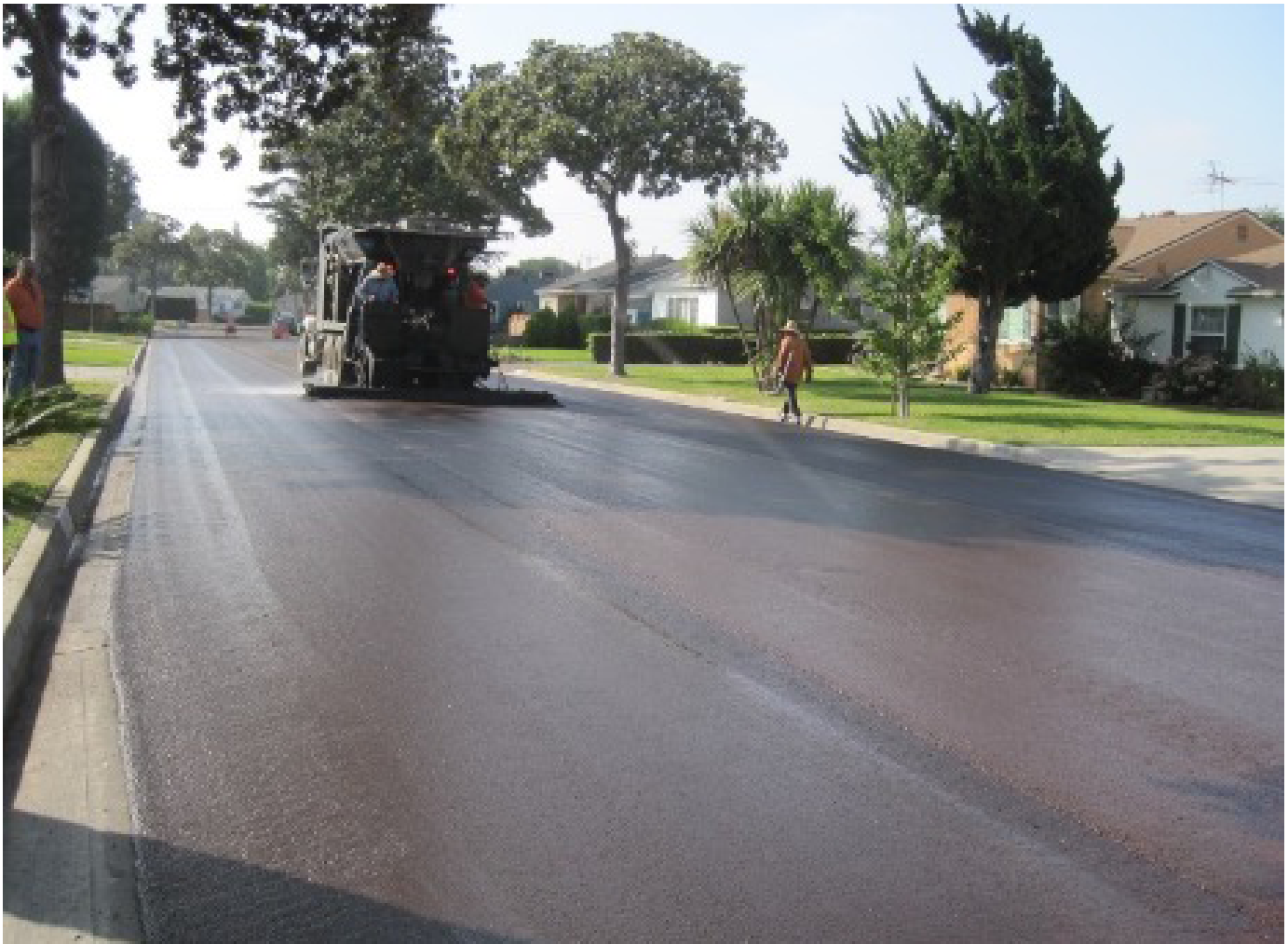
Figure 2. Typical Slurry Seal Construction
