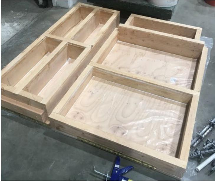
Fabricated timber mold
