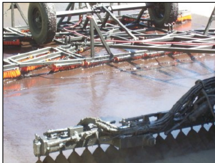
Figure 10. Scrub Seal Application
