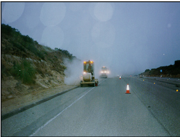
Figure 14. Sweeping Process, Shown on a Shoulder Seal
