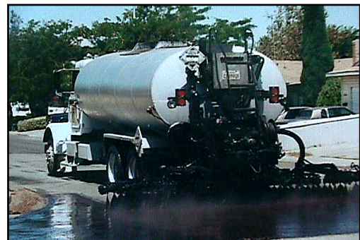
Figure 7. Spray Distributor
