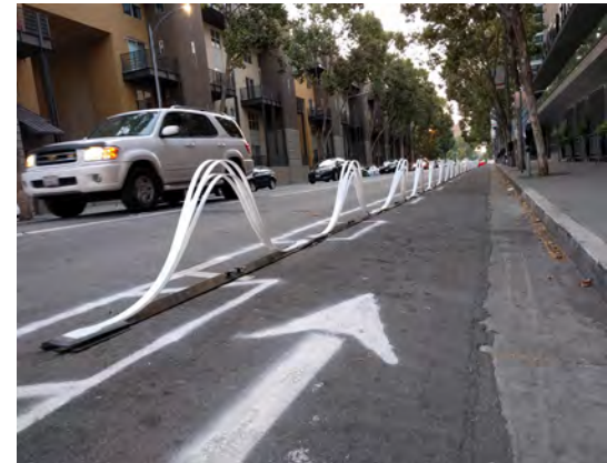
Plastic wave-shaped delineators along bikeway
