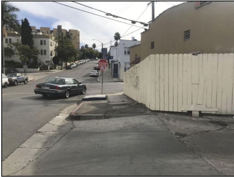
Figure 26. Cracks and Uneven Pavement
