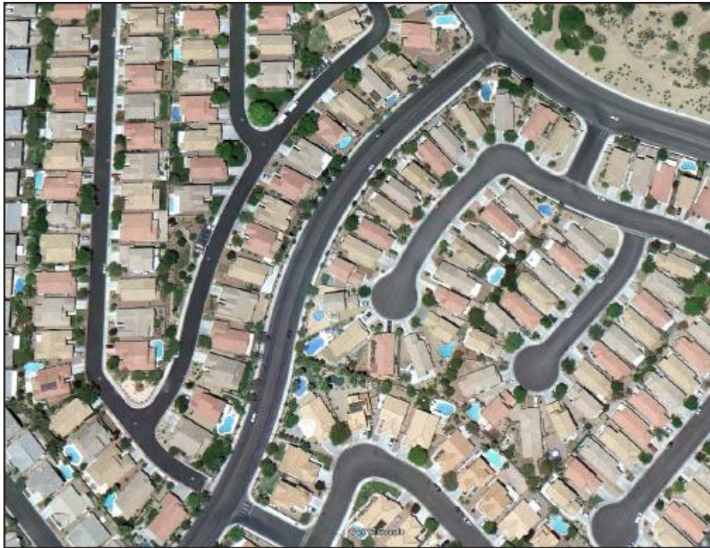
Figure 4. Private and Public Streets in Las Vegas (28 feet wide versus 37 feet wide)
