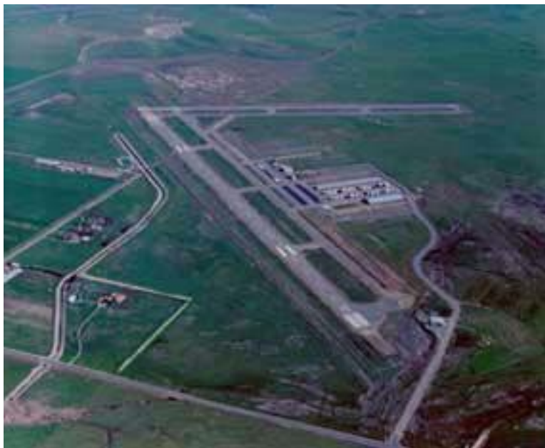
Figure 5 Byron Airport (looking south)
