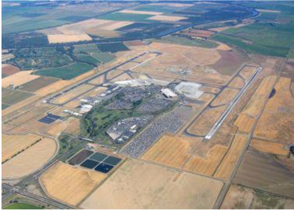
Figure 1 Sacramento International Airport
