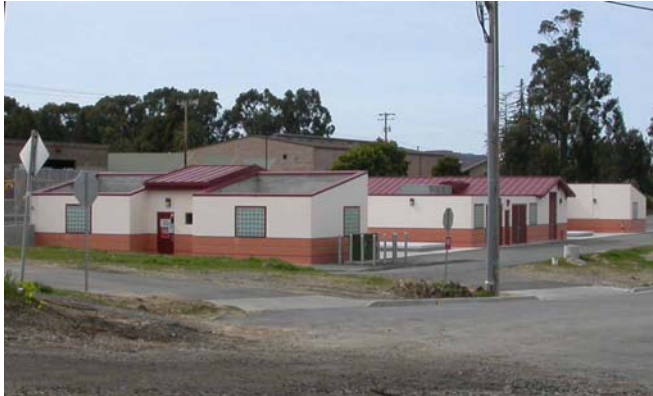
Santa Paula Vent Structure (Picture courtesy of VTA)
