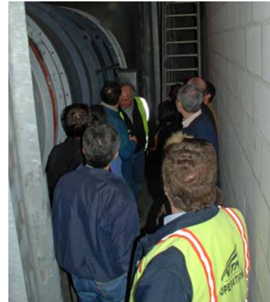
Inside the Herman vent structure (Picture courtesy of VTA)
