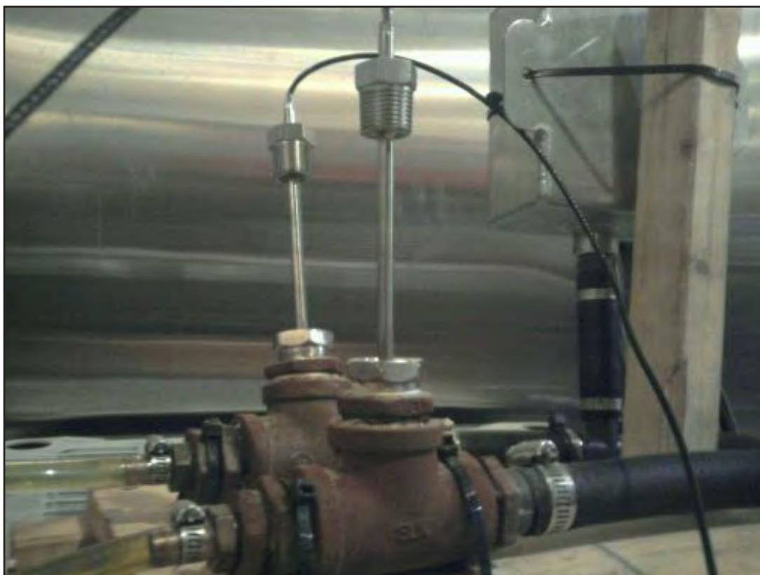
Figure 7. RTD Setup on Heat Extraction System
