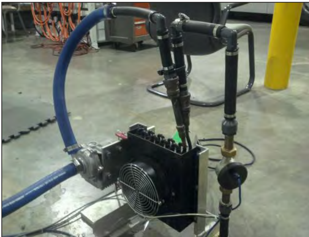
Figure 6. Heat Extraction System
