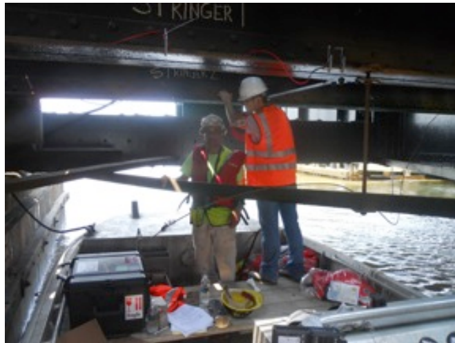
Photo 2 - Installation of various sensors on NJ Transit Bridge in Bergen County
