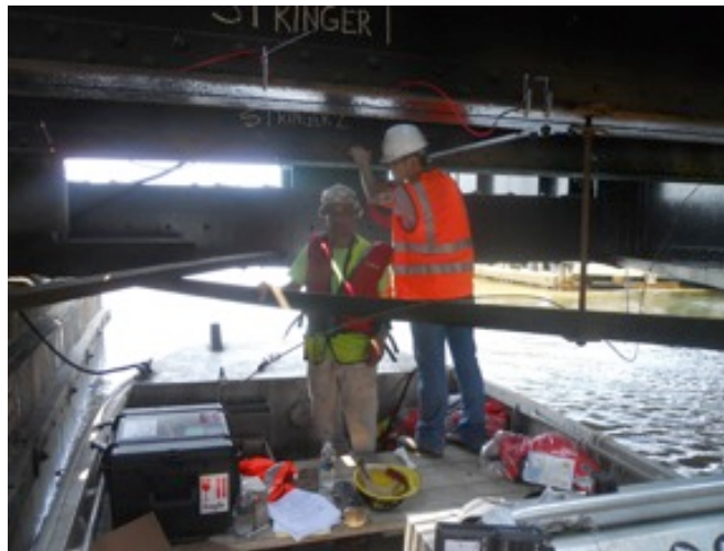
Photo 2 - Installation of various sensors on NJ Transit Bridge in Bergen County
