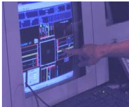
traffic control center.
